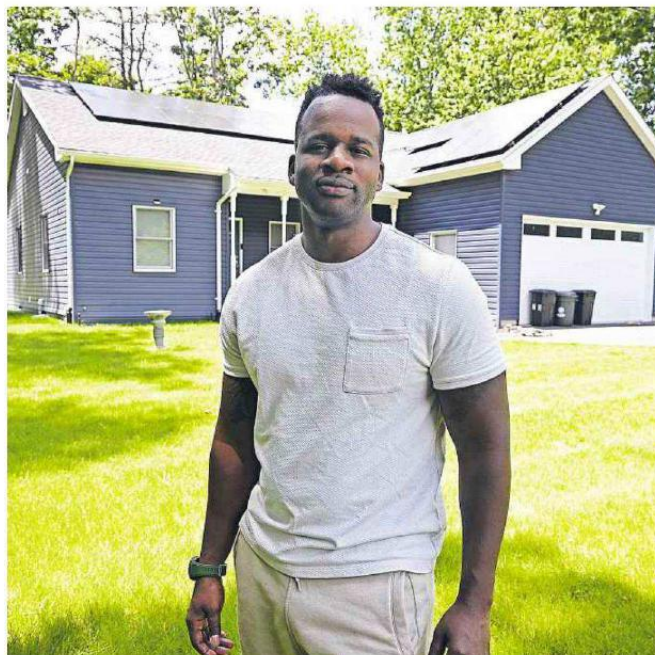
“My house is fully electric, meaning anything I need for power is run off solar,” Nasaun Lineszy said of his Middle Island home.
