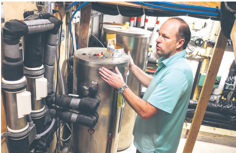
Steels with the insulated water tanks in the mechanical room in his house, which is heated and cooled by a geothermal system and also has 2-foot-deep insulated walls.
